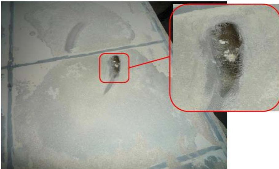
*Figure 8. The tear causing the problem*
